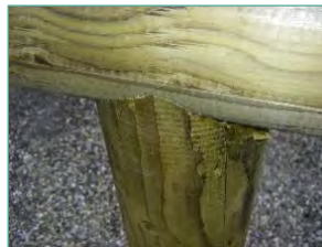
Aesthetic joint between post and rail using "tongue and groove" machining
