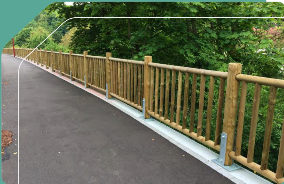
Example of hot-dip galvanised anchoring
